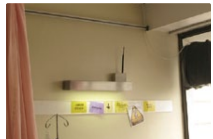
Installation of Fixed Readers at the Pilot Ward
