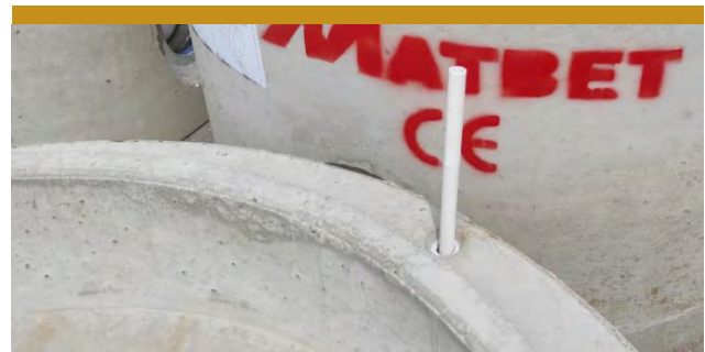
Fig. 3. An example of an RFID tag placed in a plastic tube, the so-called "antenna"
