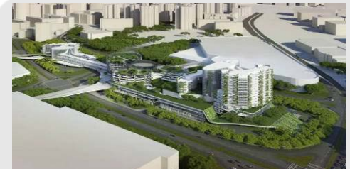
Jurong General Hospital (2014) 700-bedded regional hospital
