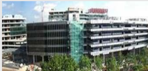
Khoo Teck Puat Hospital (2010) 550-bedded regional hospital
